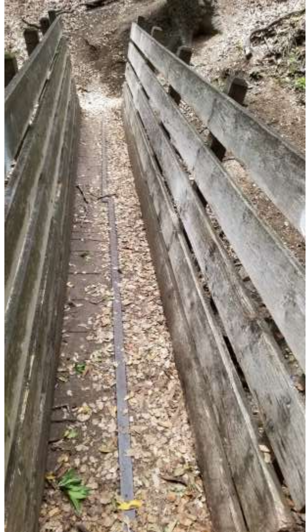
Bridge across north fork, Ziele Creek
